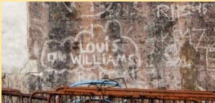
Mary Stanford Lifeboat House, Rye Grade II Listed
